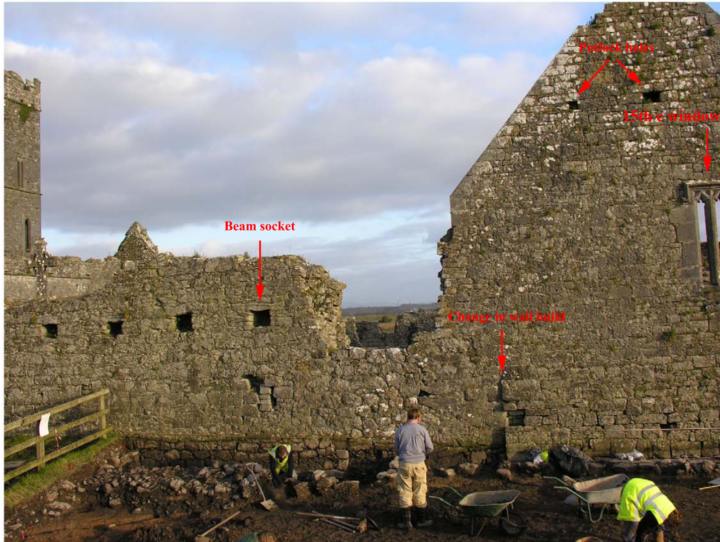
Plate 20: West wall of abbey. Looking east
