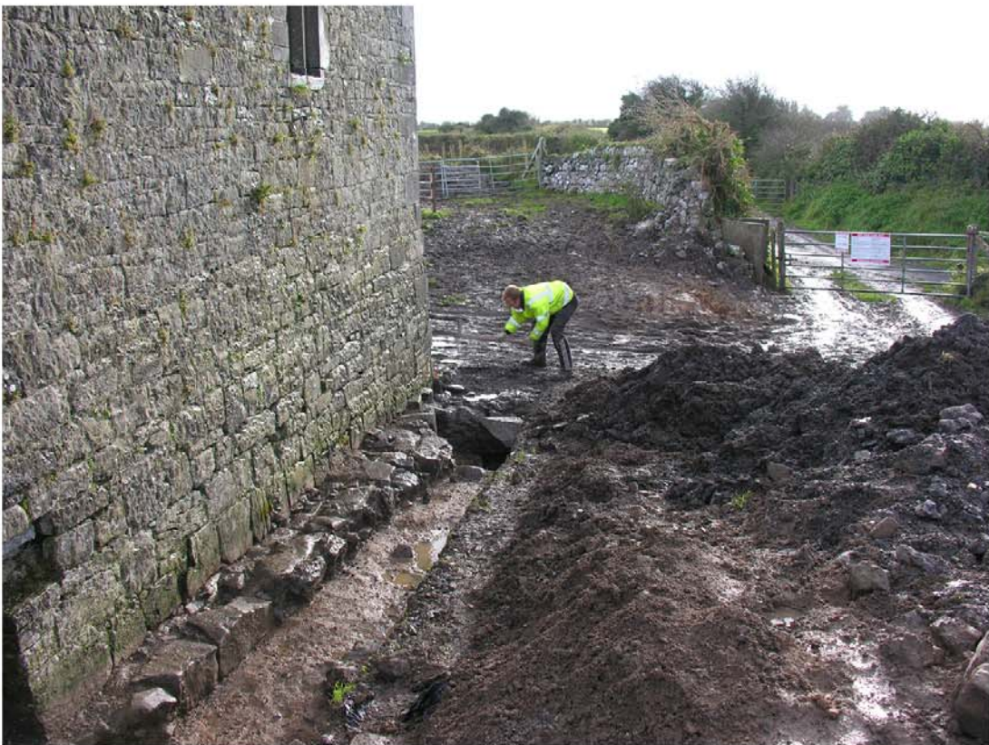
Plate 24: Foundation stones 124. Looking south-east
