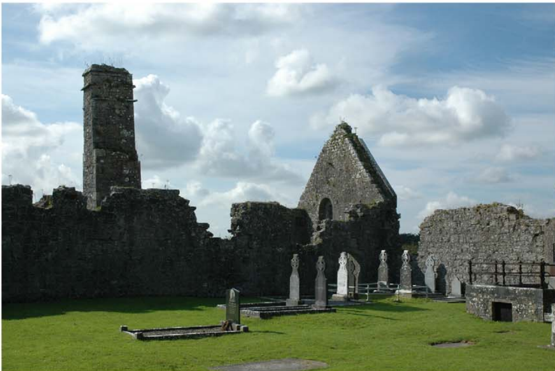
Plate 2: Cloister. Looking south-west. Kitchen at rear
