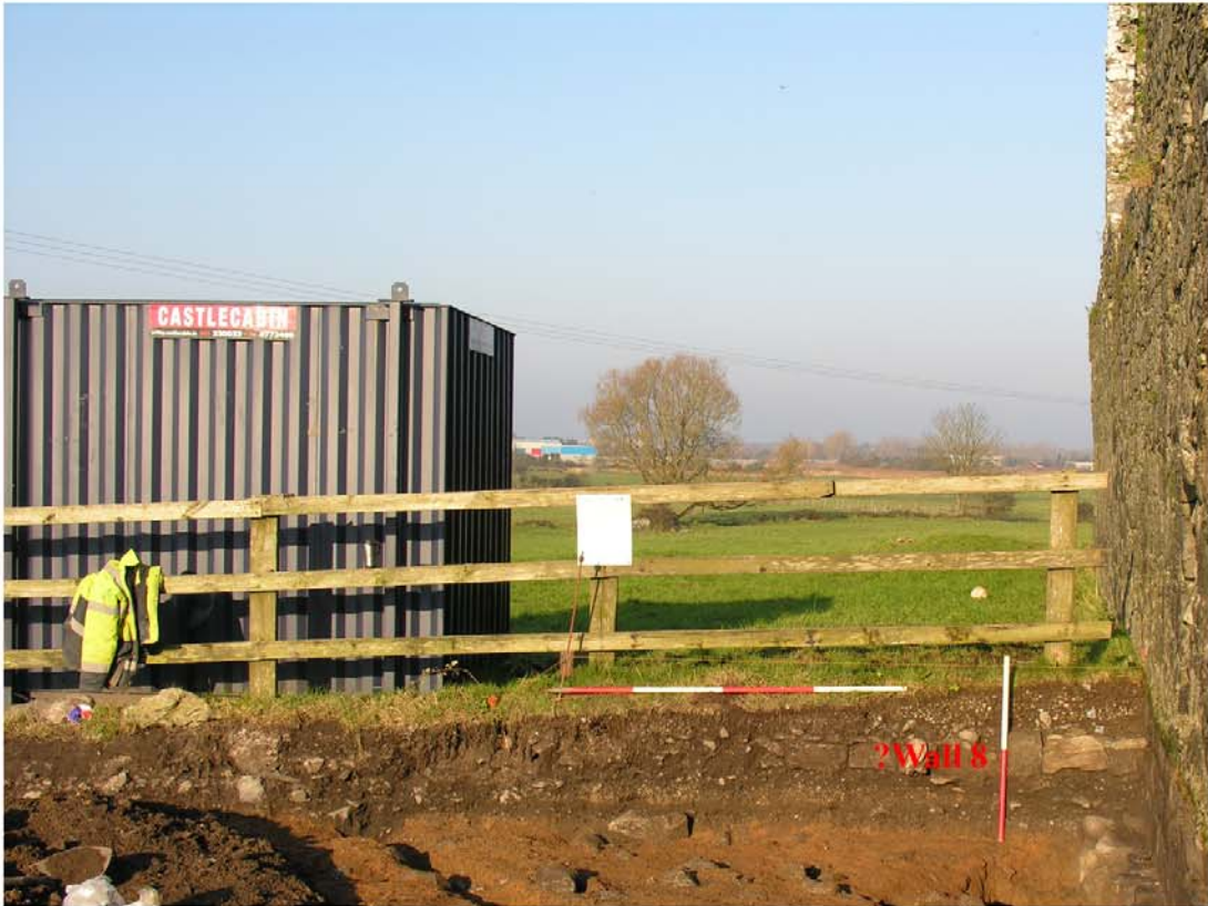
Plate 23: South-facing section showing Tumble 58 and possible Wall 8. Looking north. Scales 2m and 1m
