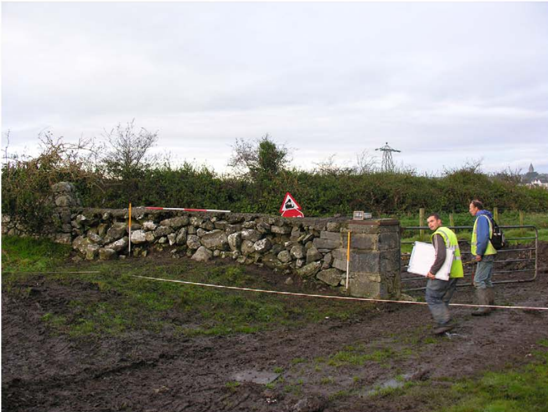
Plate 31: Wall 1. Looking south-west. Scales 2m and 1m
